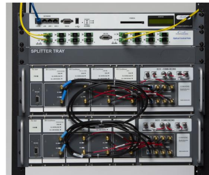
Headend: System Controller, OCH, RIU
